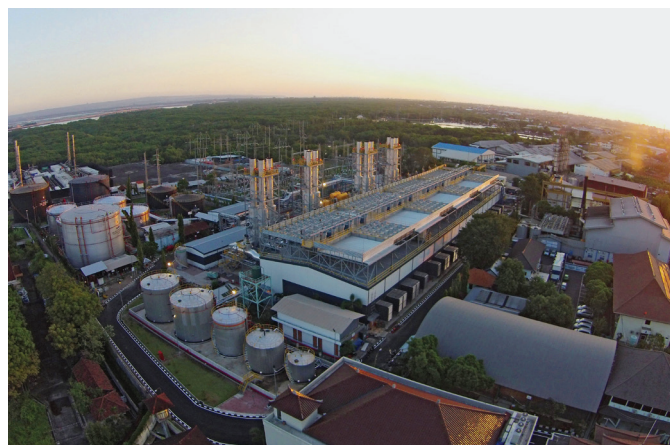
PLTDG Pesanggaran Bali 200MW plant powered by 12 Wärtsilä 50DF dual-fuel engines.
